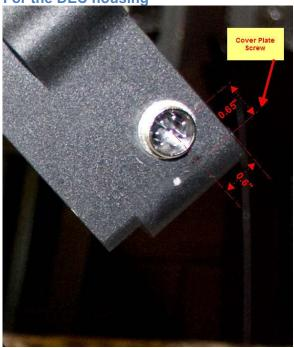
The center point for the hole is referenced with the top housing and the center point of the cover plate screw.
